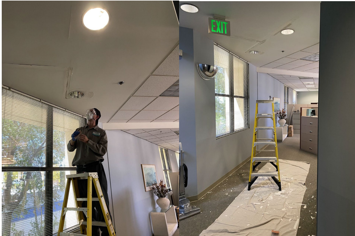
Chris Doll VCI repairing drywall
